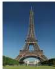
Eiffel Tower, France
